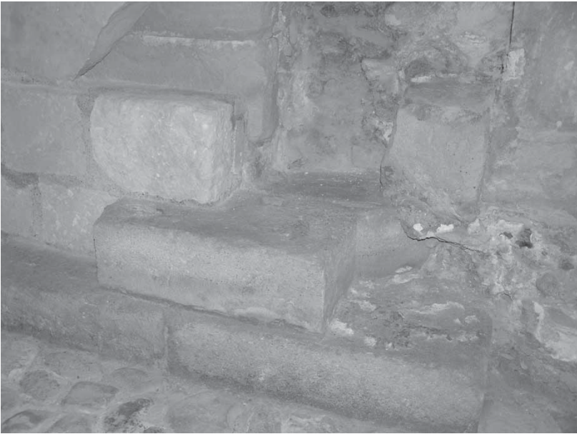
Fig. 21: Limassol Castle, cellars, south aisle, detail of wall respond plinths [M. Olympios].
